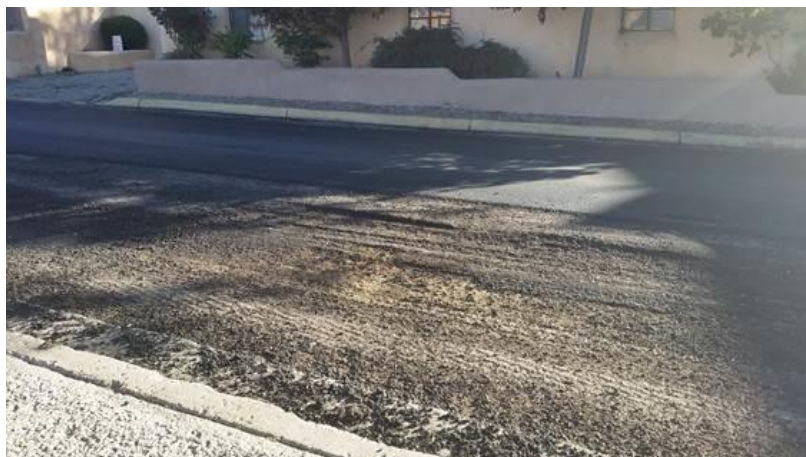
Don Fernando Street milled driving surface before paving application.
